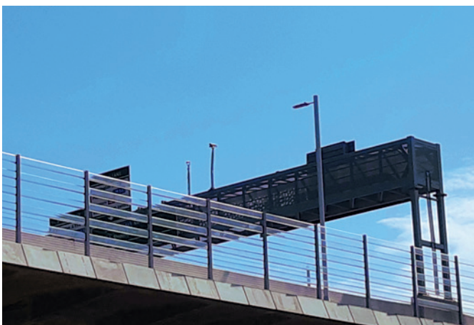
Windschutz, Mersey bridge, Liverpool PLEXIGLAS® Soundstop GS Liverpool
