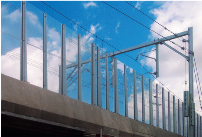
Lärmschutzwand, Parramatta Rail Link, Sydney PLEXIGLAS® Soundstop GS CC Ingal Civil Products
