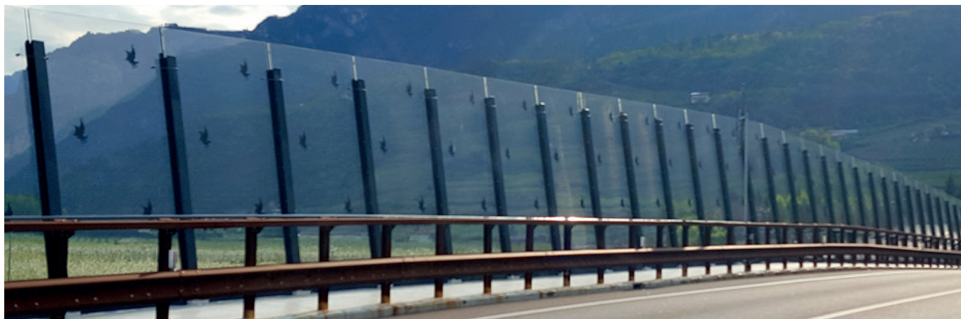
Lärmschutzwand, Autobahn Trento Sud Flyover PLEXIGLAS® Soundstop GS CC 20 mm, Clear Trento Sud Flyover
